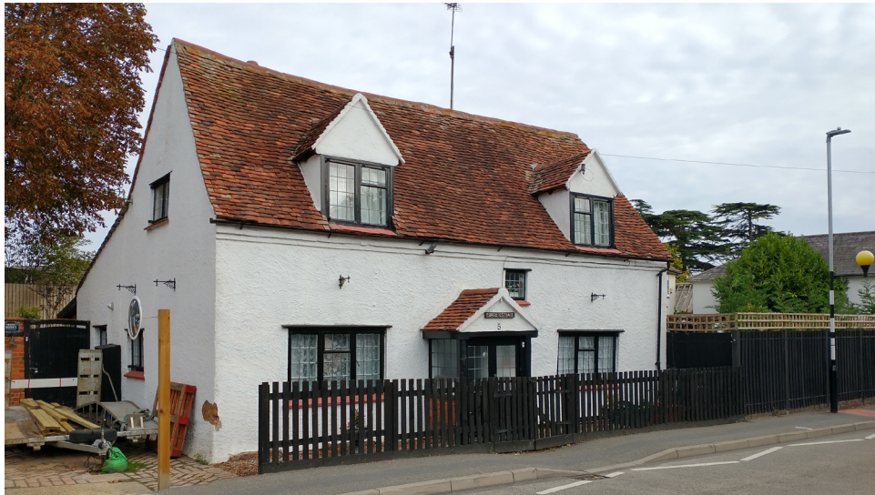
Figure 8 Grade II listed Forge Cottage on Valley Road which has been dated to the sixteenth century or earlier
